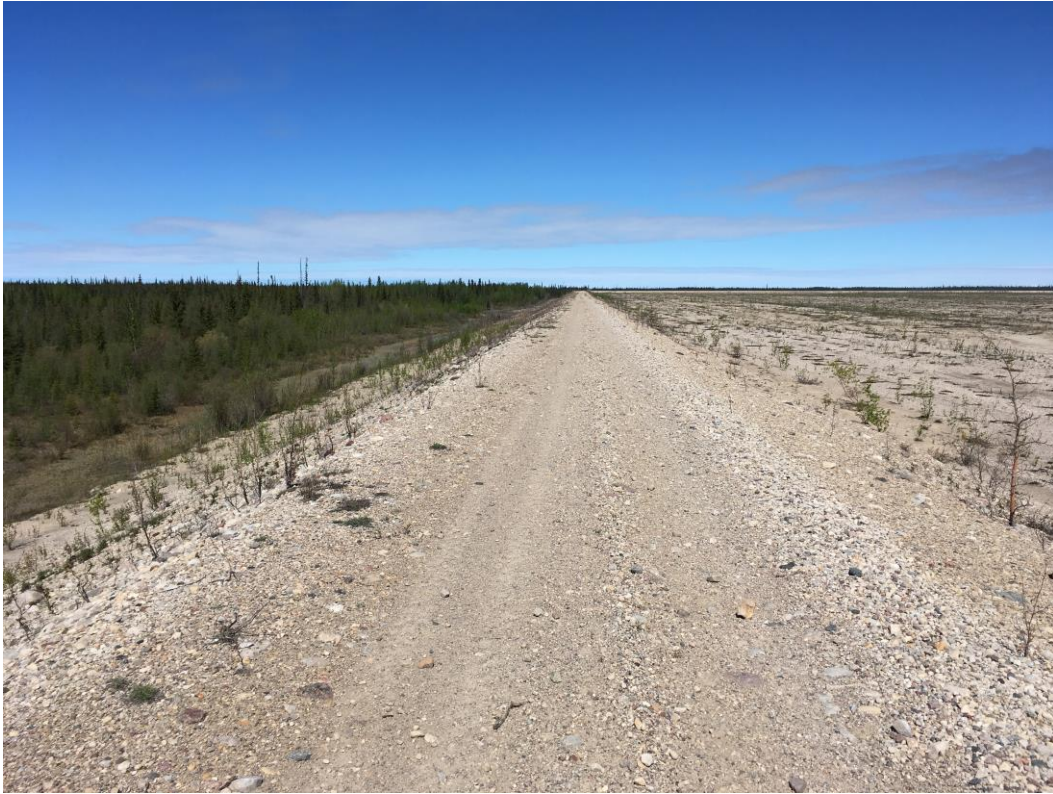
West Dyke, Central Area, Facing North
