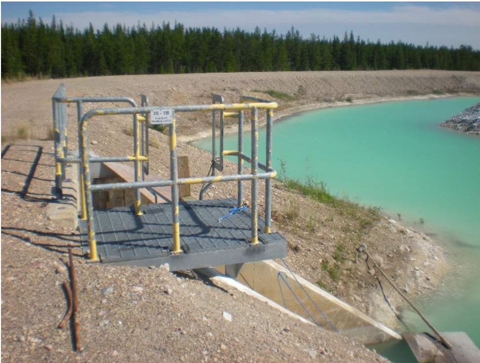
Photograph 13: Settlement Pond Spillway (Spillway No.2) – Settling Pond Side. 27 July 2017
