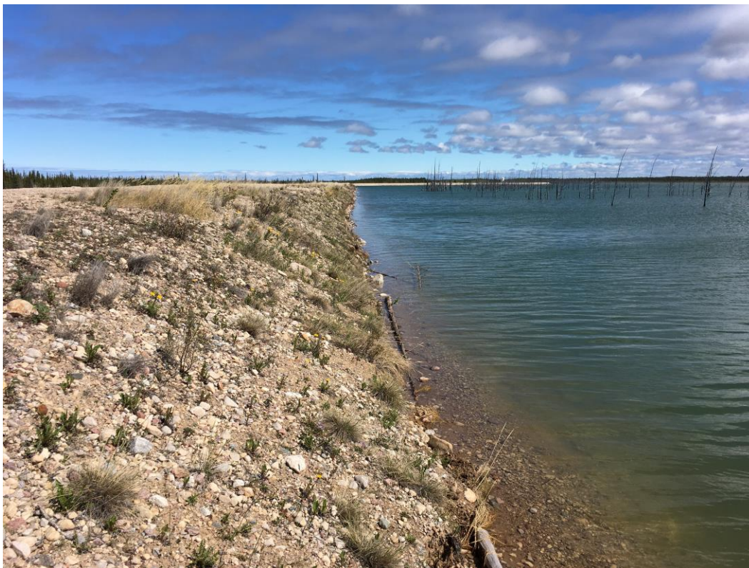
North Dyke, 2008 Construction area, mine waste side, facing East
