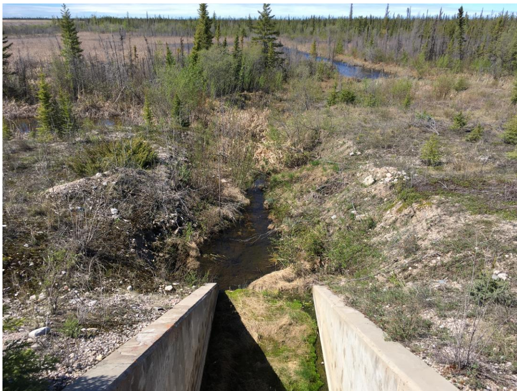
Downstream Main Pond Spillway.
