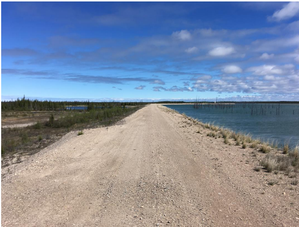
North Dyke, 2008 Construction area, facing East
