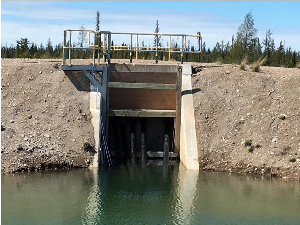
Treatment Pond Spillway, Upstream Side.
