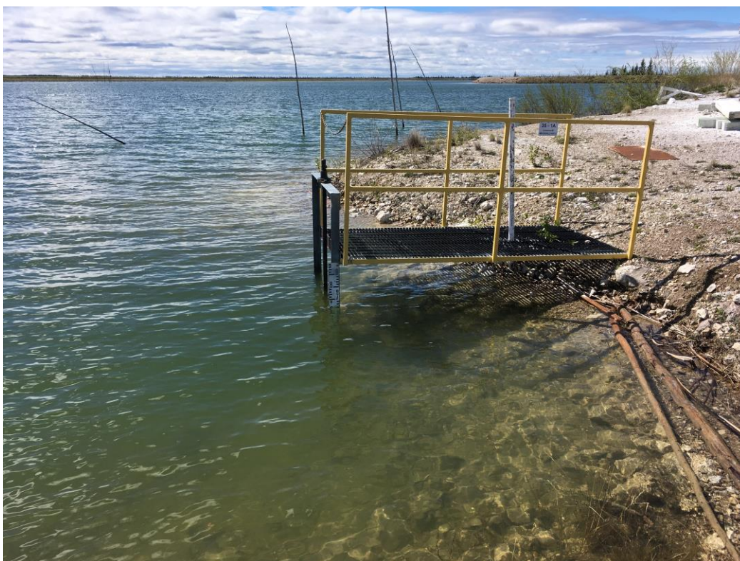
Main Pond Culvert to polishing pond.
