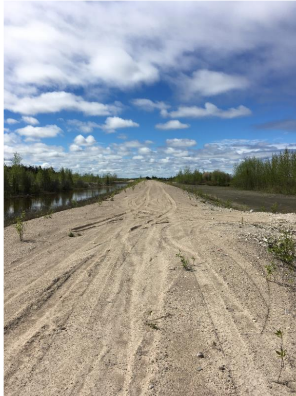
South Dyke East End, facing west
