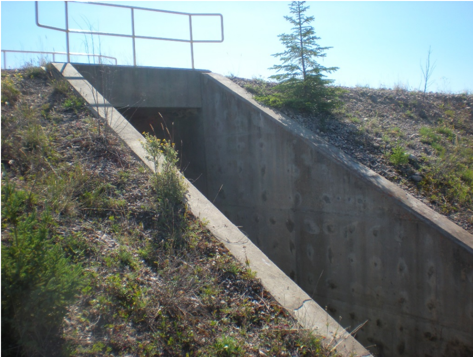
Photograph 11a: Main Pond Spillway (Spillway No. 1). 27 July 2017
