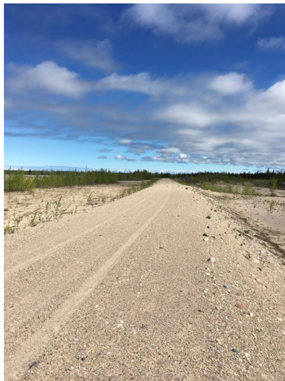
South Dyke East End, facing east
