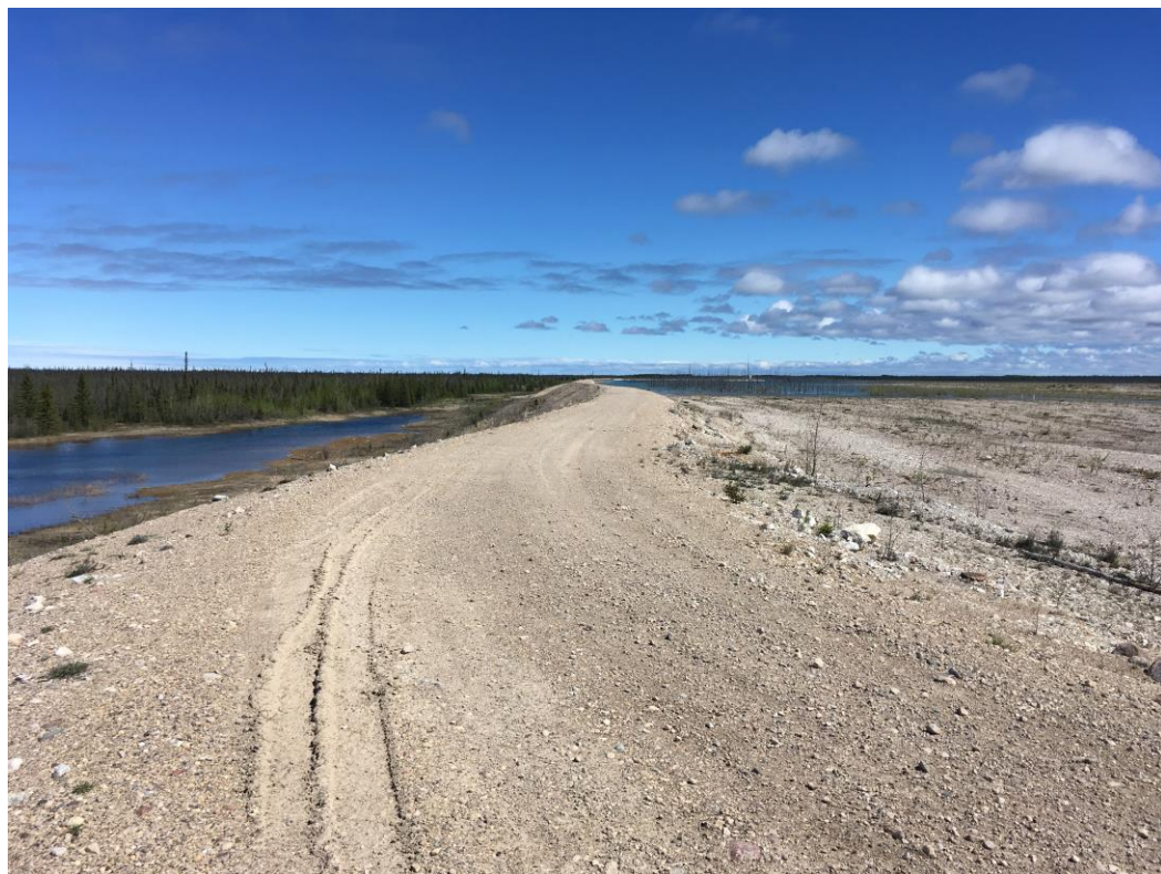
North Dyke, facing East.
