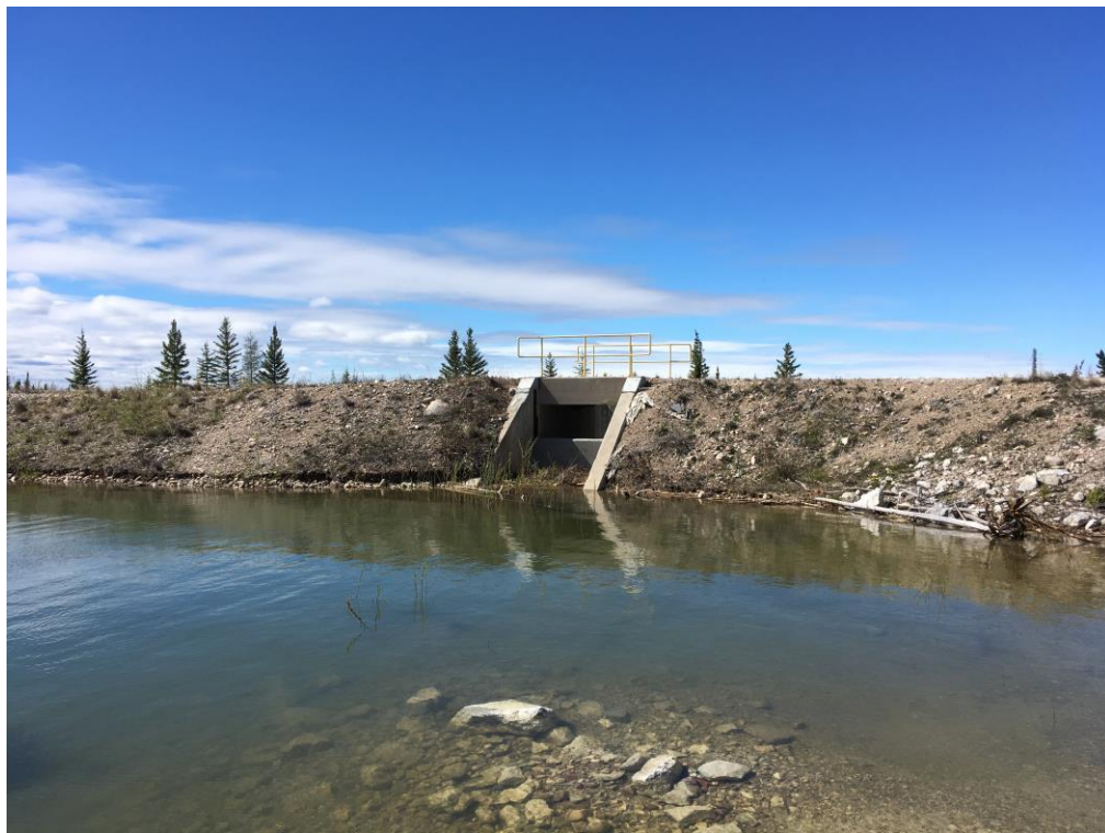
Main Pond Spillway, Mine Waste Side
