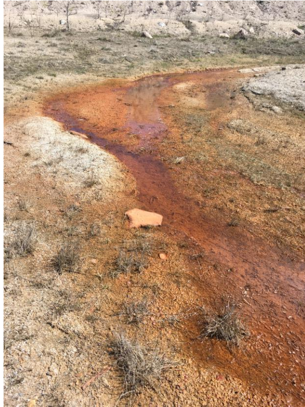
West Dyke, Previously Observed Boil Area, Staining near toe, facing East.
