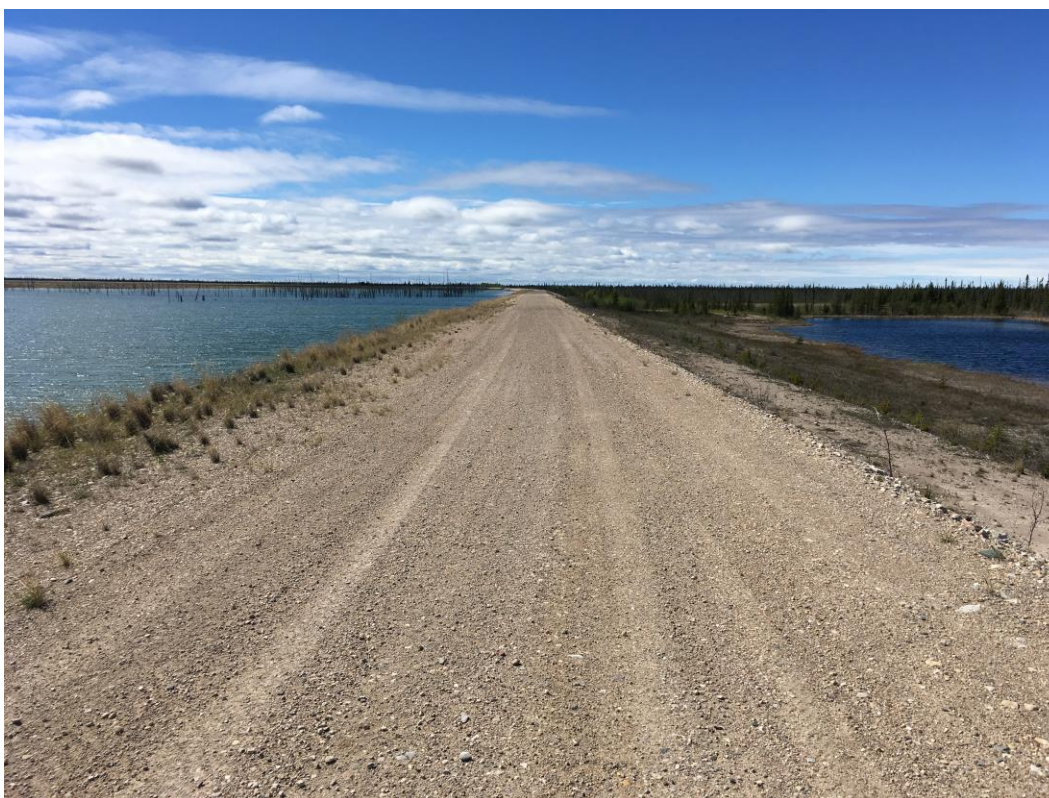
North Dyke, 2008 Construction area, facing West.
