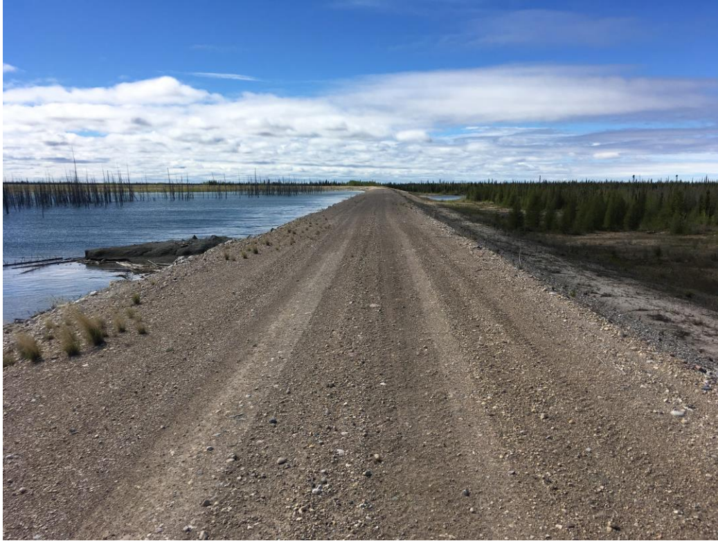
North dyke central area facing west
