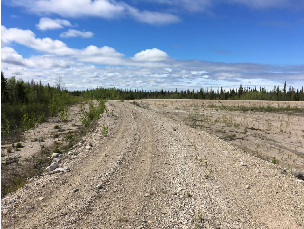
South Dyke, West End corner, facing West.
