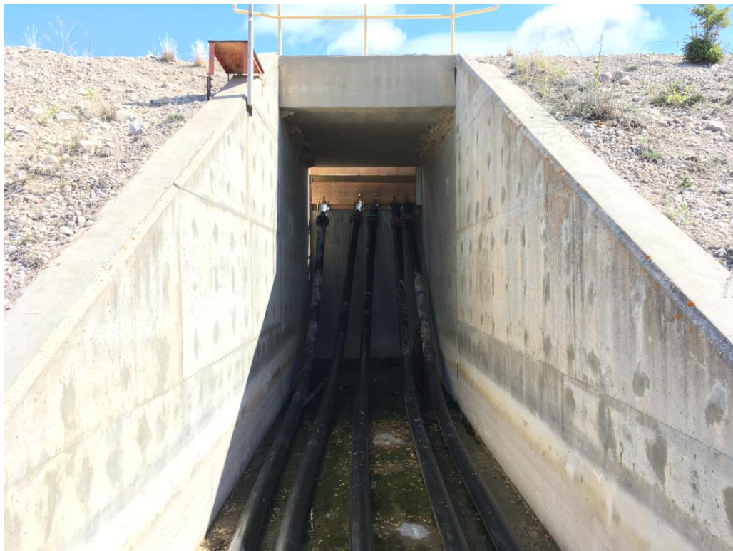
Downstream side of treatment pond spillway.
