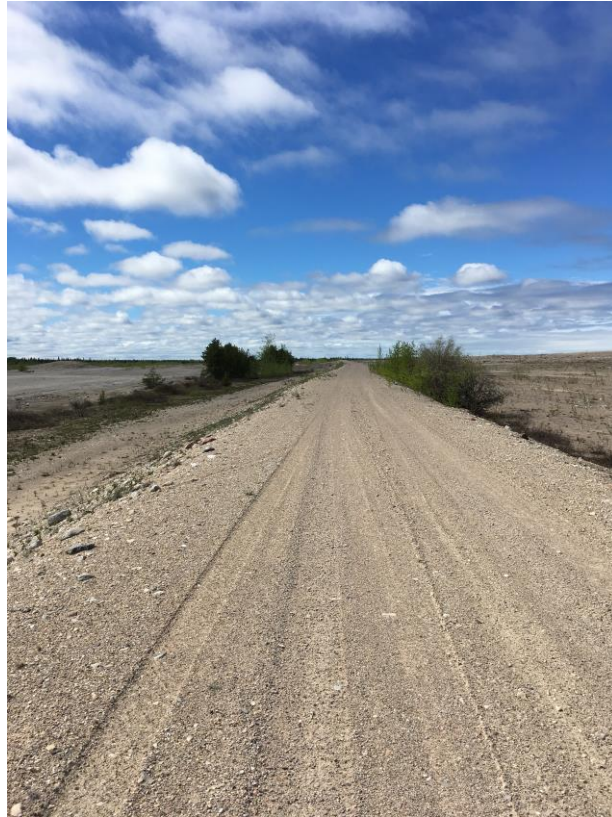
South Dyke, approaching central area facing west.
