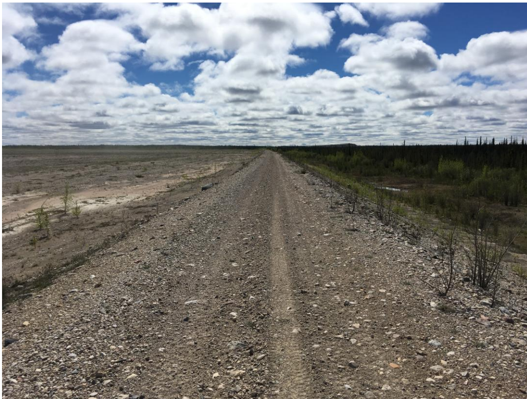
West Dyke, Central Area, Facing South
