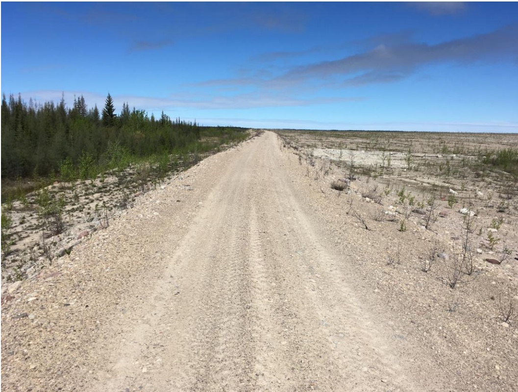
West Dyke, South end, facing North
