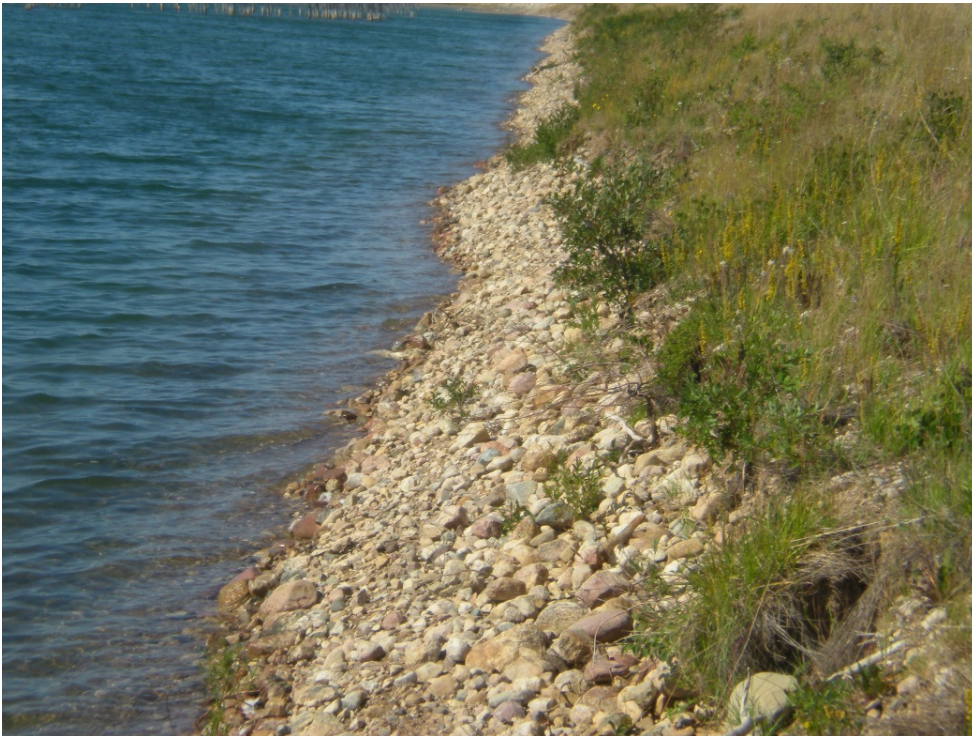
Photograph 10a: North Dyke Upstream Face, Gravel and Cobbles at Pond Waterline. 27 July 2017
