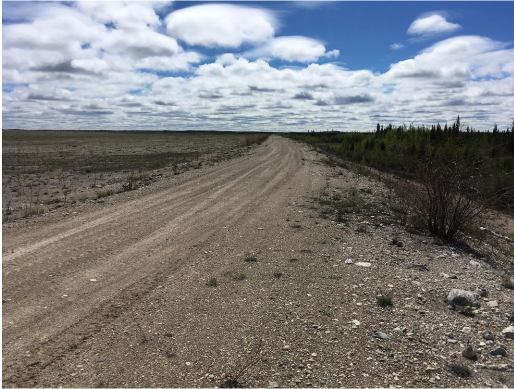
West end of North Dyke, facing South, mine waste side.
