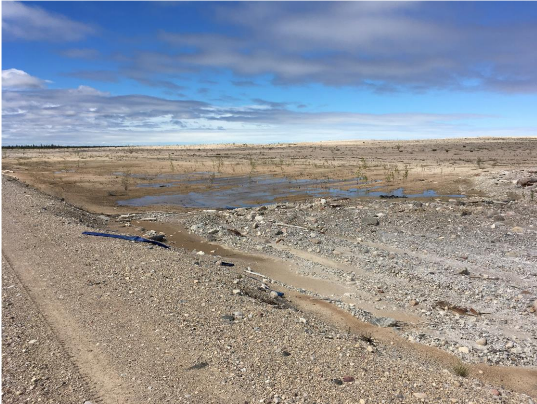
South Dyke, Central Area, minor seasonal water upstream side
