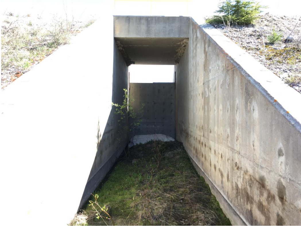
Downstream side of main pond spillway
