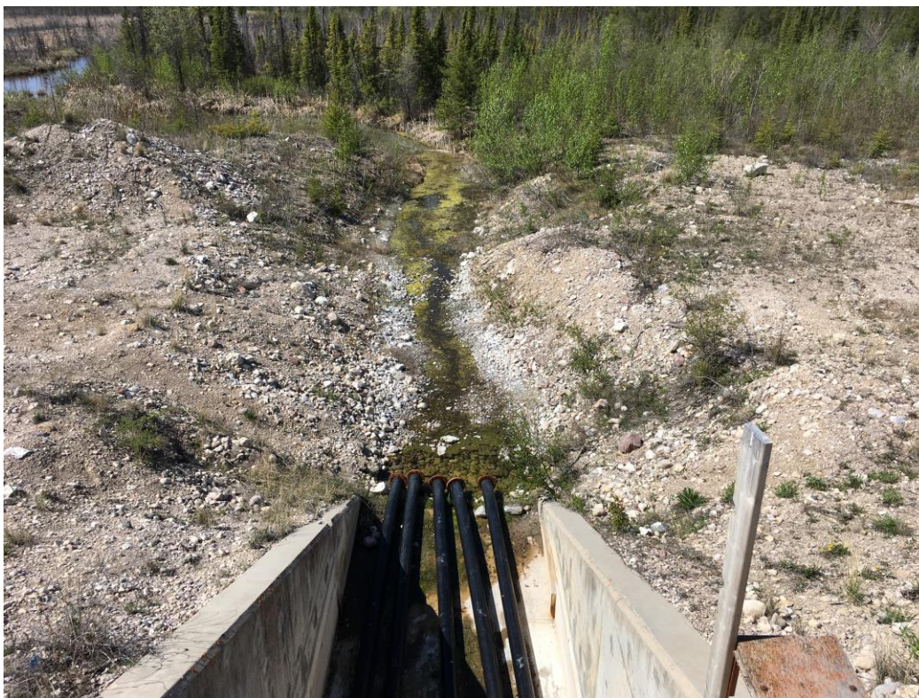
Treatment Pond Spillway, Down Stream Side.
