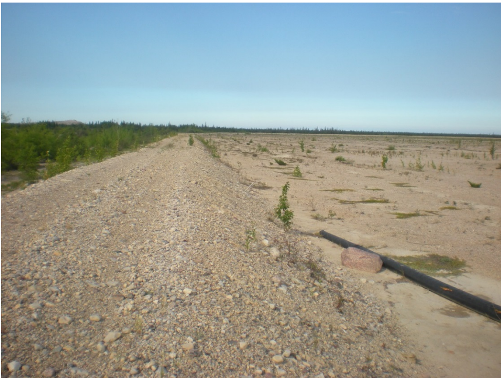
Photograph 2: South Dyke – Upstream Face of Central Portion, Looking West. 27 July 2017
