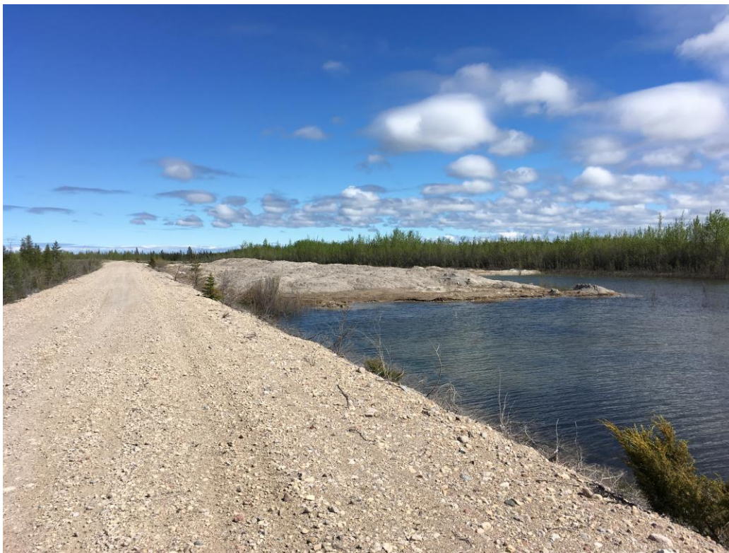
North Dyke, East of Polishing Pond
