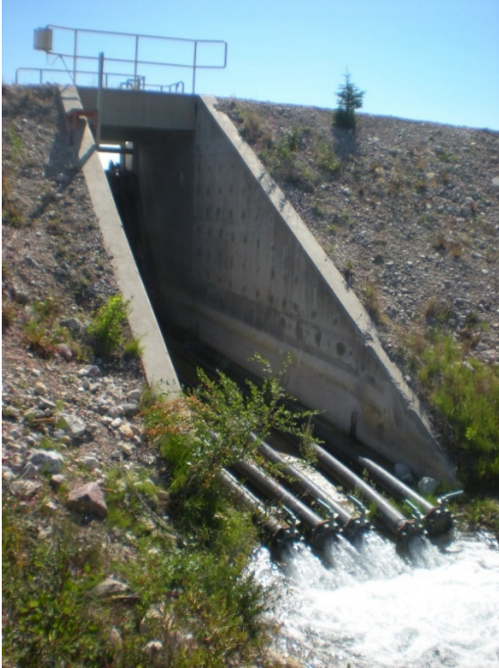
Photograph 12: Settlement Pond Spillway (Spillway No.2) – Syphon Piping Discharge at Outlet. 27 July 2017
