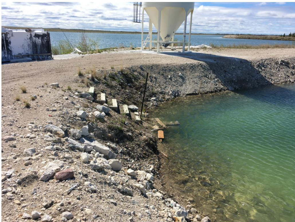
Main pond to polishing pond culvert, polishing pond side
