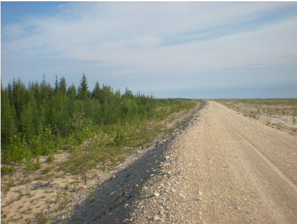
Photograph 4: West Dyke – Downstream Face, Looking North. 27 July 2017
