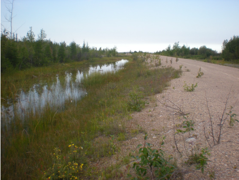
Photograph 1: South Dyke – Downstream Face at East End, Looking West. 27 July 2017
